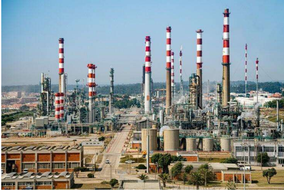
Figure 3 - Refinery view from entrance
