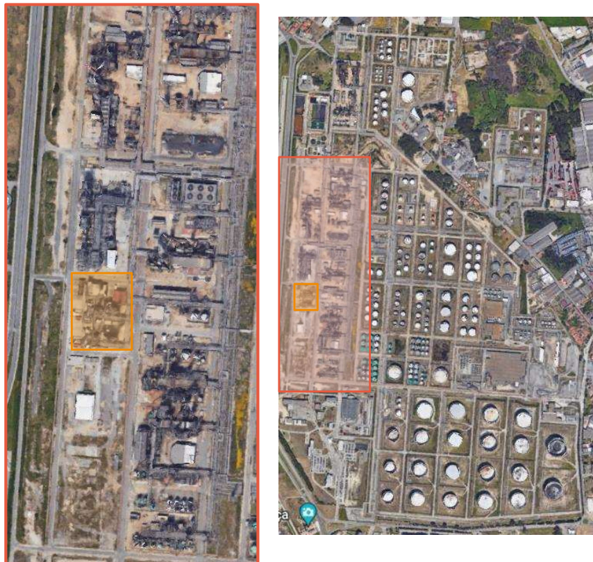
Figure 4 – Refinery plant and location of the COGEN unit
